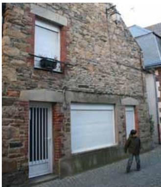
Percement inadapté, menuiseries PVC
